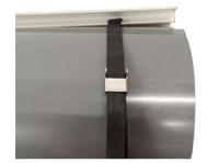
Use the tightening tool and start tightening
